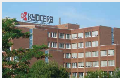
Sales & Technical Center (Germany)
