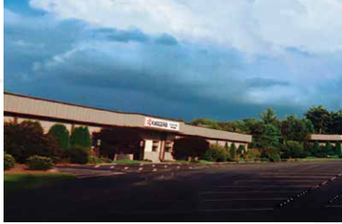
North Carolina Facility (USA)
