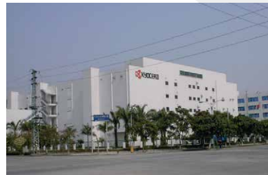
Silong Facility (CHINA)
