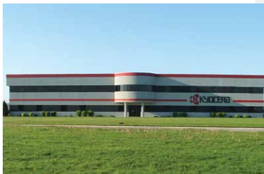
Ohio Facility (USA)
