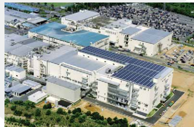
Yokaichi Facility (JAPAN)
